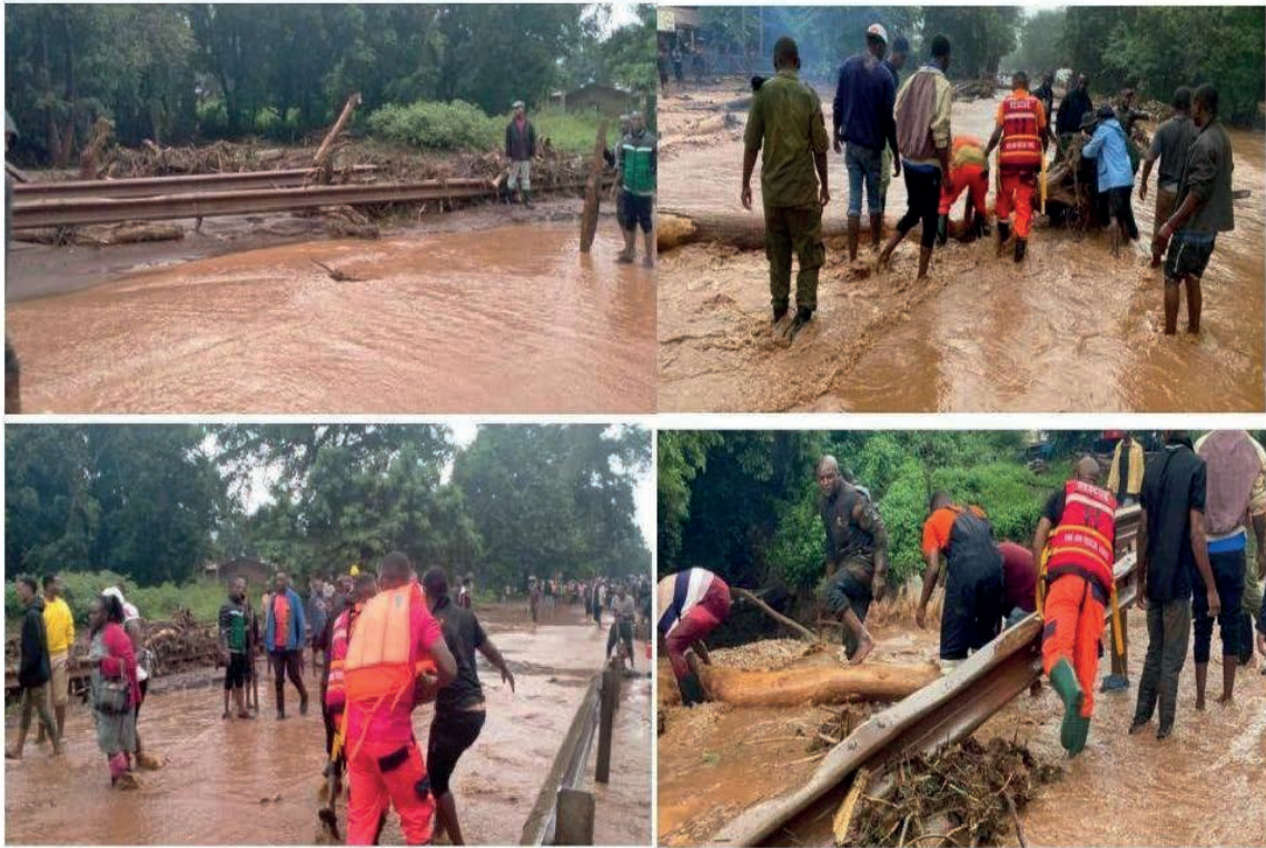
Figure 13: Flooding of Moshi-Arusha-Dar es Salaam highway road. Regional fire and rescue services removing logs on the road in Kiboriloni area, in Kilimanjaro region on 06th May 2025 (Source: https://www.mwananchi.co.tz/mw/habari/kitaifa/watu-17-wamenusurika-kusombwa-na-maji-mkoani-kilimanjaro-5030182 ).
